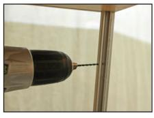
Step 2. Drill hole at each ends for light bar clips. (Drill 3rd hole in center of rail for 6' showcase)
