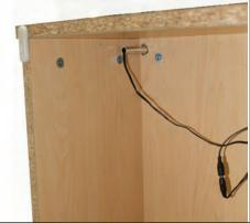
**Step 11.** From bottom of showcase, connect power cord to power supply.
