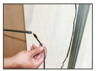
**Step 7.** Feed power cord through aluminum pole.
